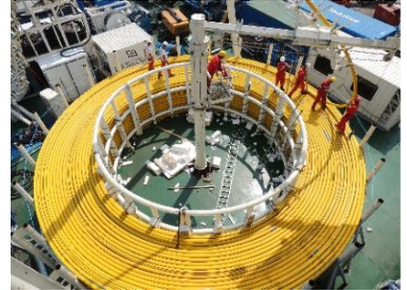
LD TRAVOCEAN has been awarded by EDF of the contract for the installation of the main DC cable, and has proposed a specific lay and burial spread dedicated to the shallow water area and high current working zone. Cable protection has been done with the burial on the 1st 5 km and Articulated Pipes protection installation on 10 km taking into account the specific soil conditions of the area which is crossing several types of seabed.
