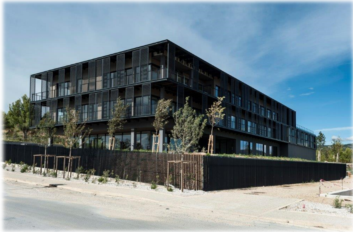
BATIMENT / BUILDING LOUIS DREYFUS TRAVOCEAN
